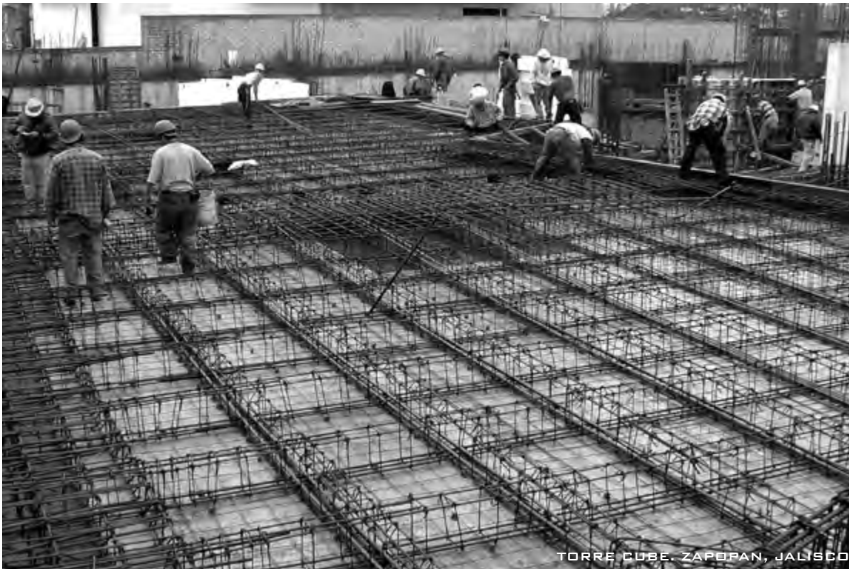
PISO INDUSTRIAL NAVE ECOPARK. ZAPOPAN, JALISCO.
