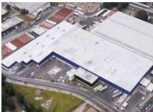
NAVE INDUSTRIAL EMERSON
