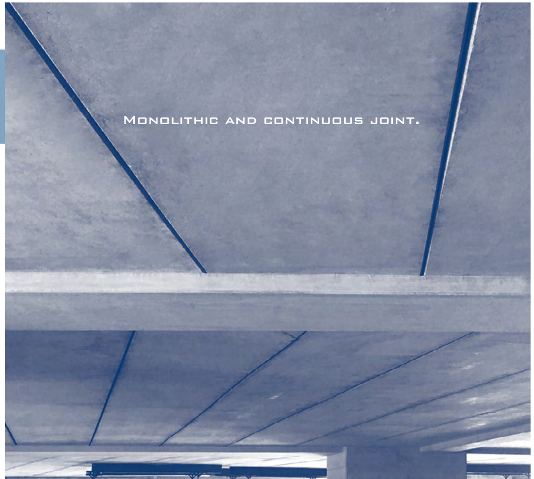
DETAIL OF UNION BY PRESLAB-BEAM
