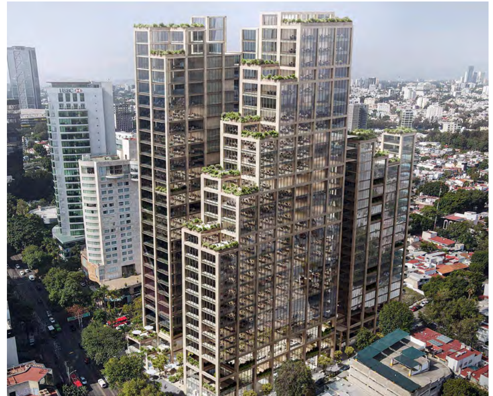
TORRE THE DISTRICT
